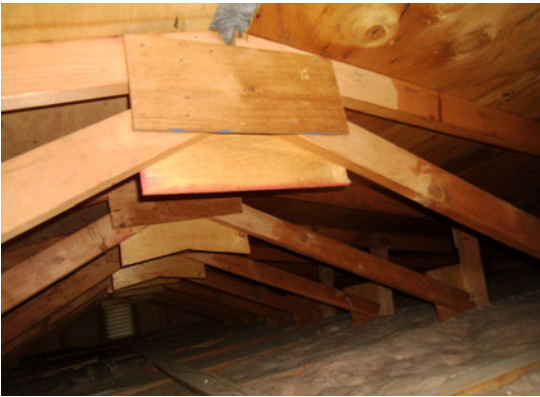
Home made trusses in garage
