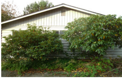
Vegetation on structure
